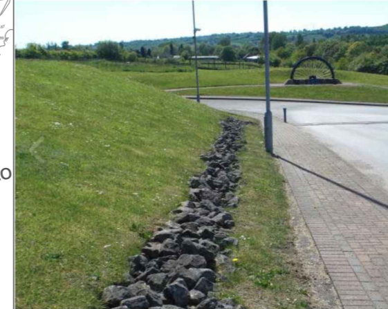
Proposed filter trench will drain runoff from shared private drives where possible.
